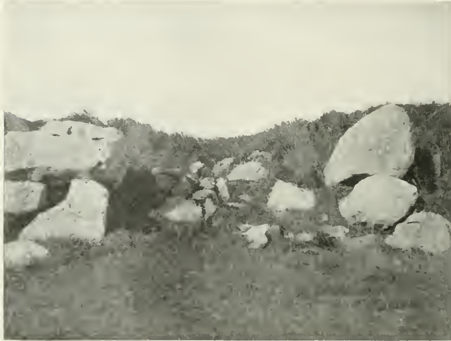
FIGURE 1. — A POSTERN ON THE WEST SIDE OF LA CIVITA No. 6 on the Plan. Width, 2.85 m.
